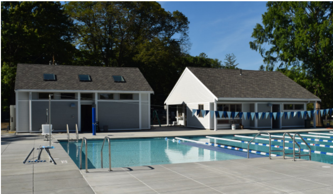
Typical Pool Building Construction: Wood framed, cedar or fiber-cement clapboard siding, asphalt shingle roofing, fiberglass windows and doors. Photo also illustrates concrete pool deck and its finish.
