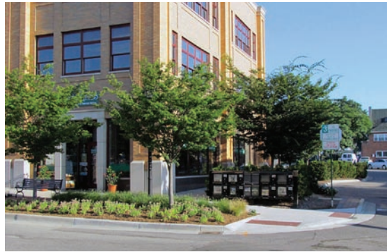
Bump outs provide space for amenities and improve connections for pedestrians Northville, MI Photo: Dan Burden
