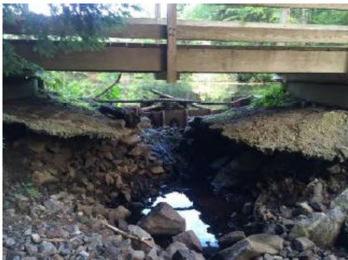
The Coffin Pond Spillway which was rated as “Not Passable” during the Fish Passage Assessment. Photo Credit: Stantec.
