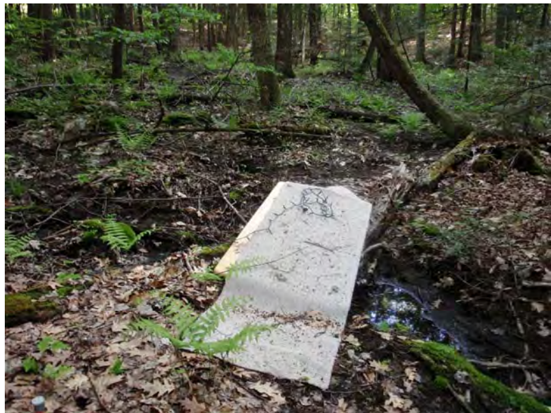
materials in easement at drainage in southern section.JPG
