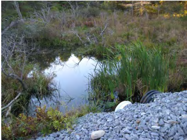
Culvert and wetland, approx 150 yds from entrance gate
