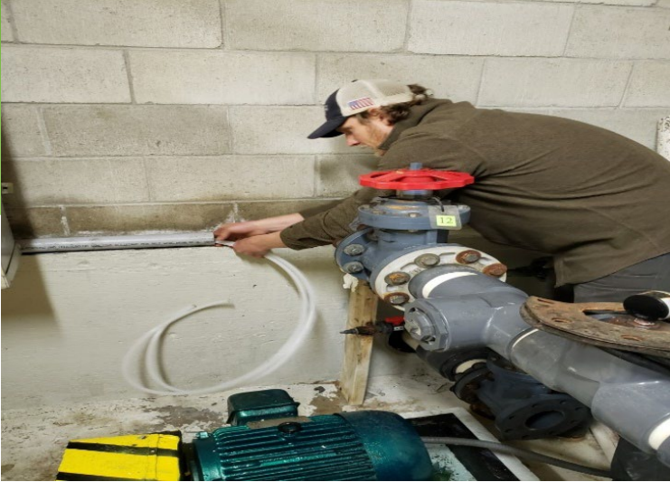
Chlorine Line Replacement at Coffin Pond
