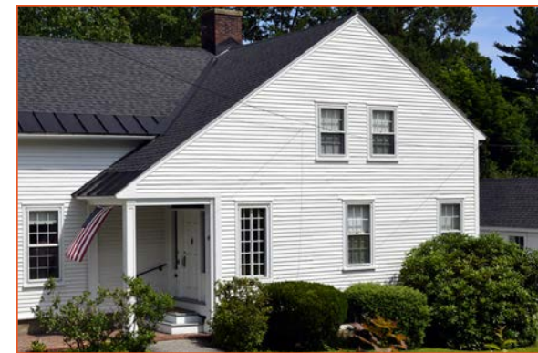
This home on Federal Street is an example of wood clapboards aligning cleanly with the top and bottom edge of the windows.
