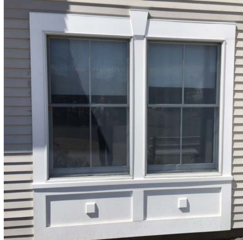
After (work done 2015)
