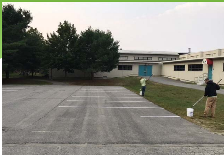
Parking lot maintenance
