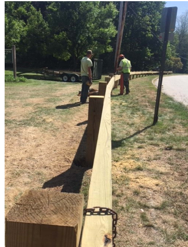
Guardrail Replacement
