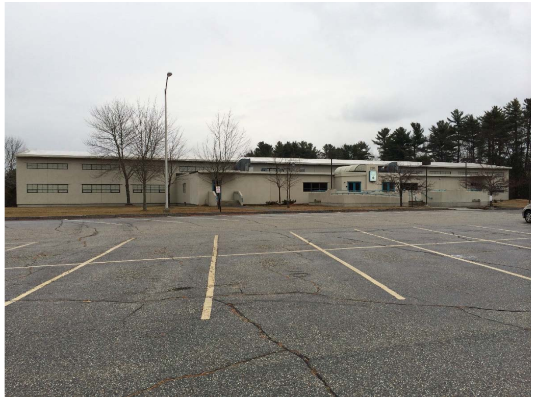
Pavement Repairs and Re-Striping
