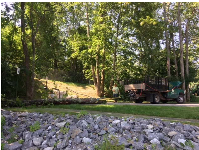
Downed trees and debris removal
