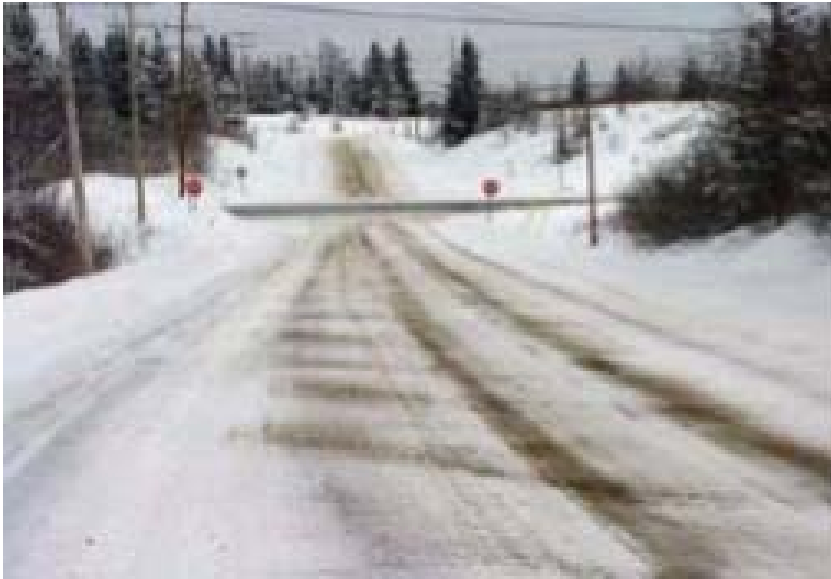
Roadway Treated with Sand/Salt Mix
