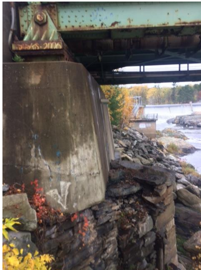
3.9 Existing Brunswick abutment looking west
