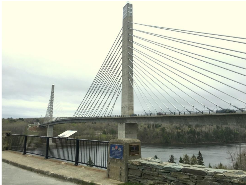
3.19 Repurposed old abutment for bridge memorialization Penobscot Narrows Bridge, Prospect, Maine
