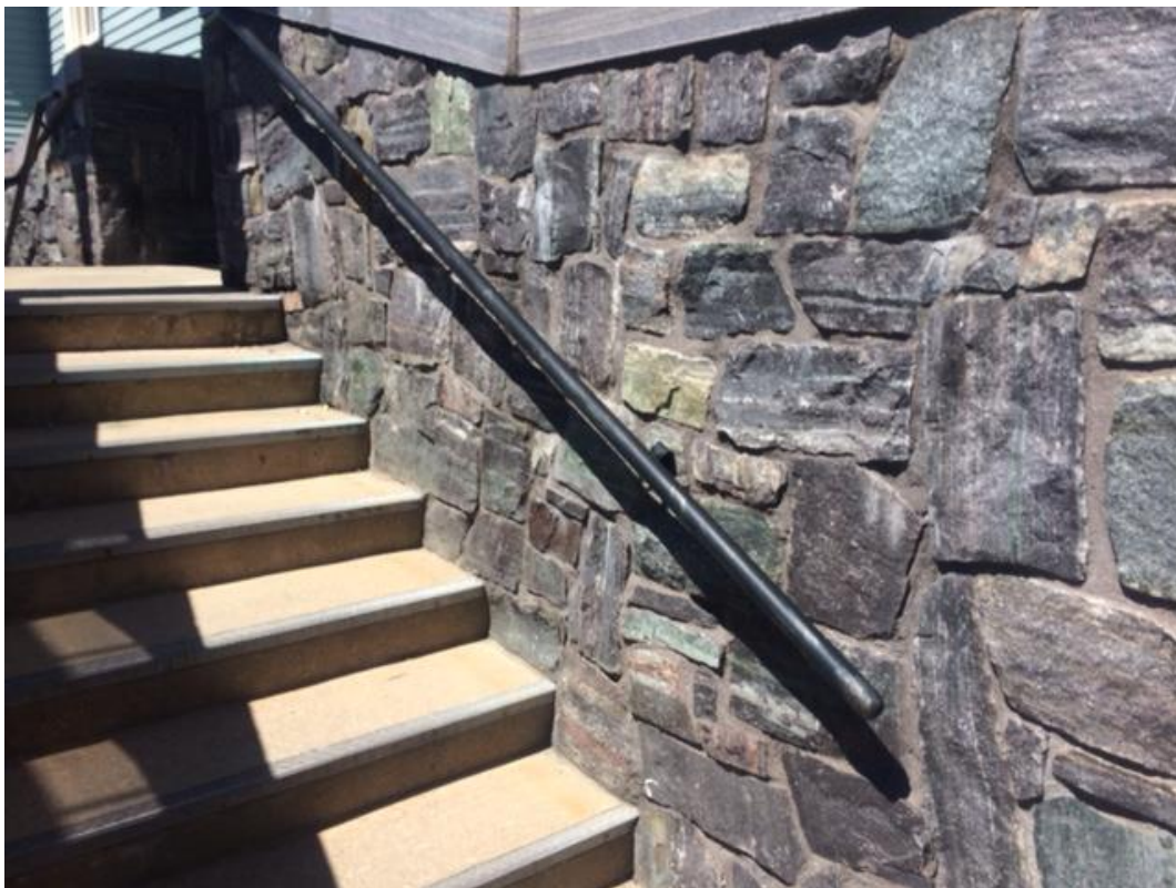
5.5 Wall materials, handrail and stairs, York Public Library
