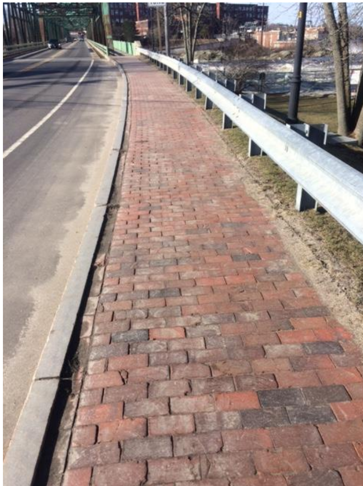
5.2 Existing westerly sidewalk approaching Frank Wood Bridge, Topsham
