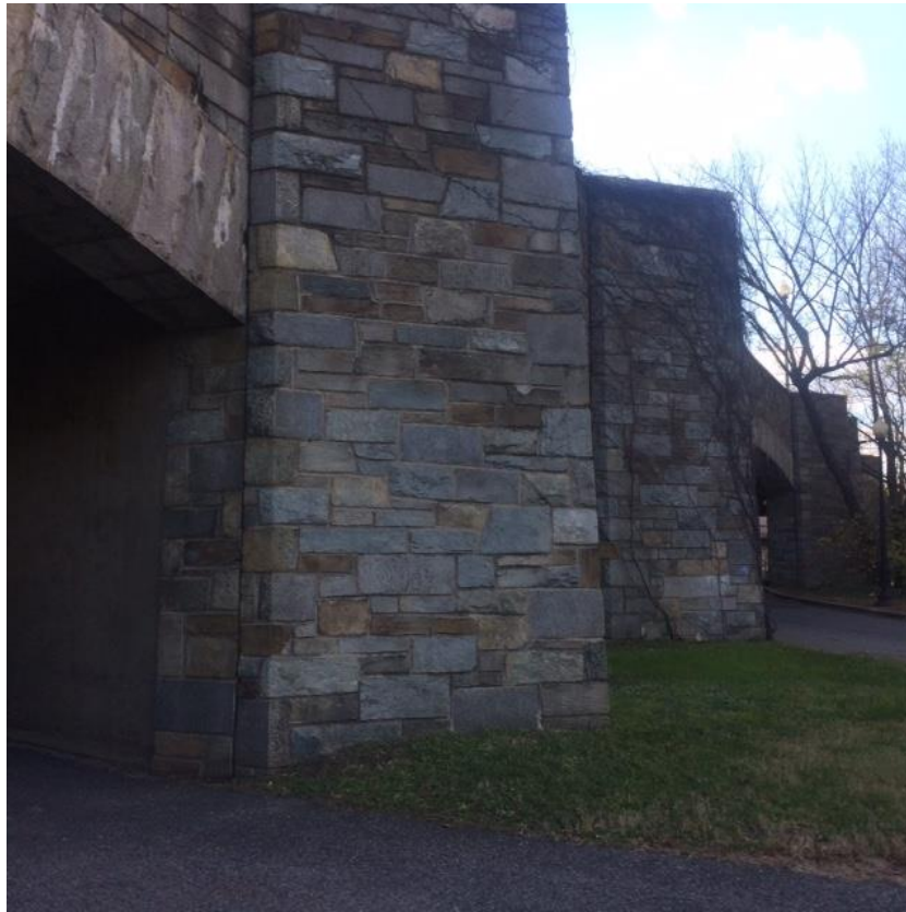
5.4 Bridge abutment, Washington, DC
