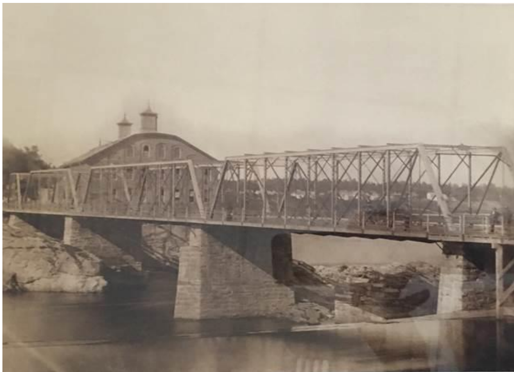
4.5 Bridge at this site previous to Frank J. Wood Bridge Trapezoidal granite block pier with pointed upstream end
