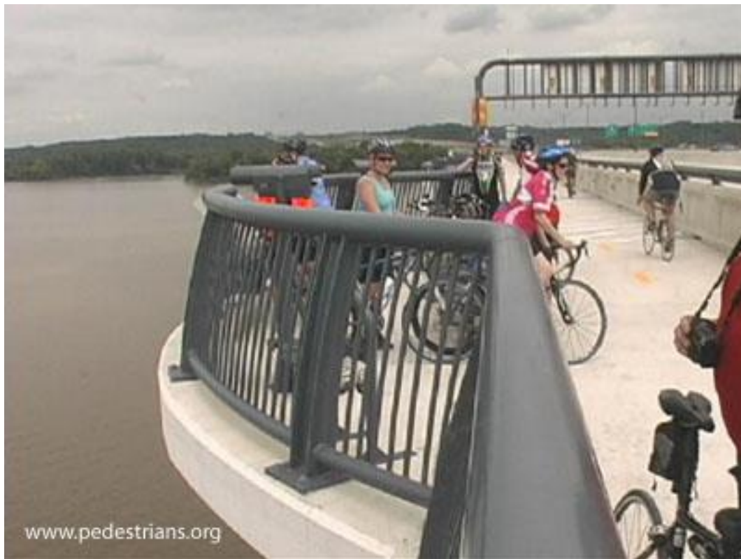
3.2 Crescent-shaped pedestrian bumpout on Woodrow Wilson Bridge over the Potomac River, VA & MD
