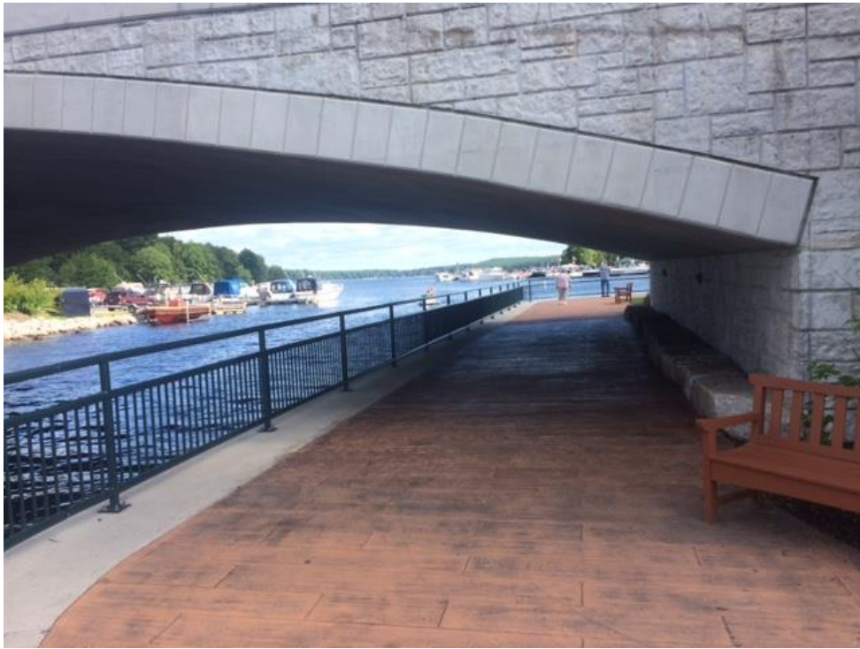
3.17 Pedestrian underpass example: Naples Causeway, Maine
