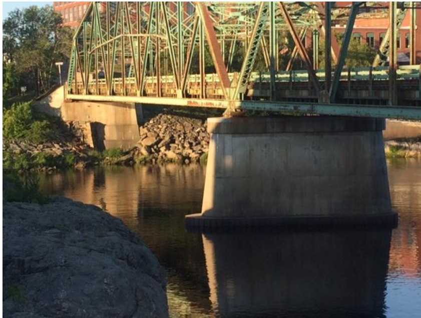
4.2 Frank J. Wood Bridge pier
