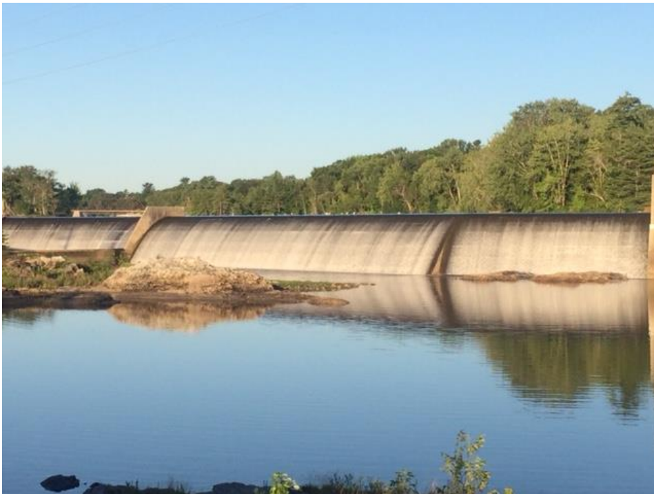
3.12a View upstream to Swinging Bridge from Topsham Overlook
