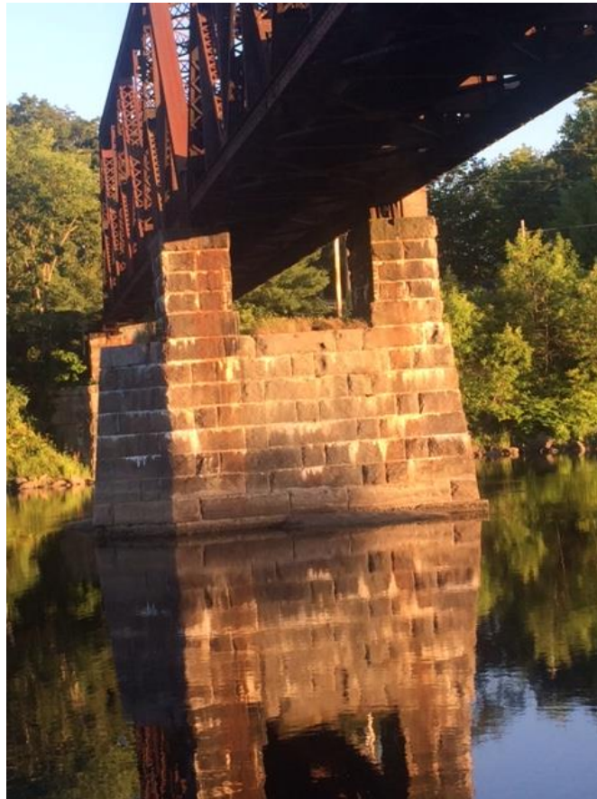
4.3 Black Bridge carrying railroad (Mill St. to Bridge St.)
