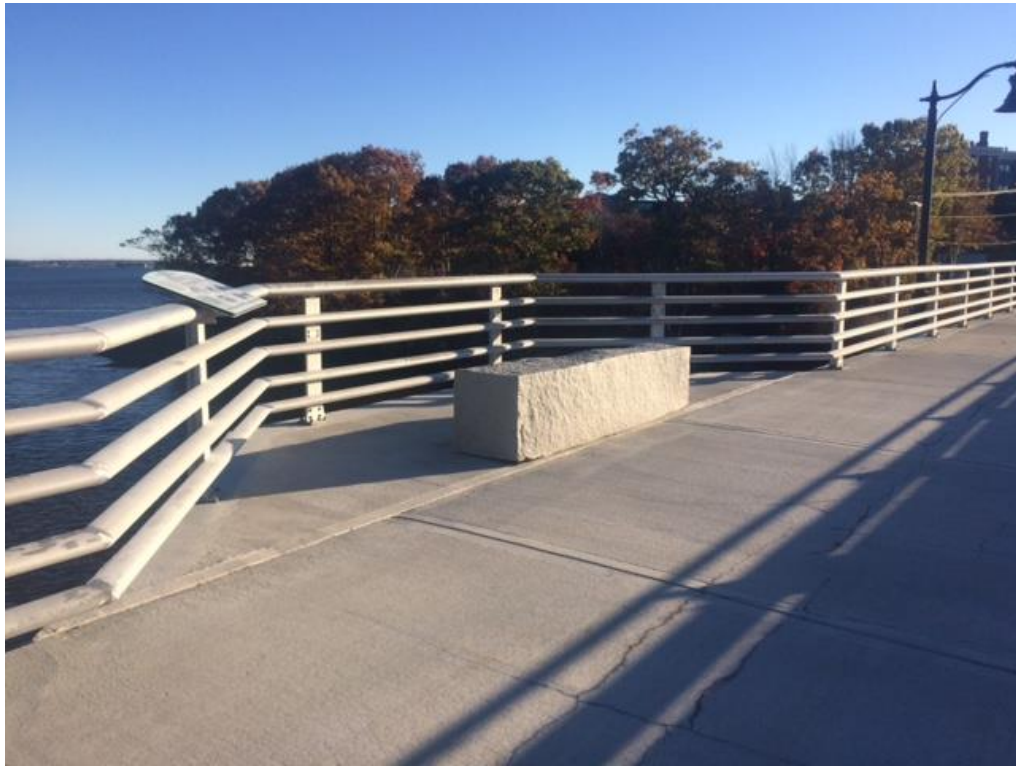
3.3 Seating in bumpout at Martin's Point Bridge, Portland & Falmouth, Maine
