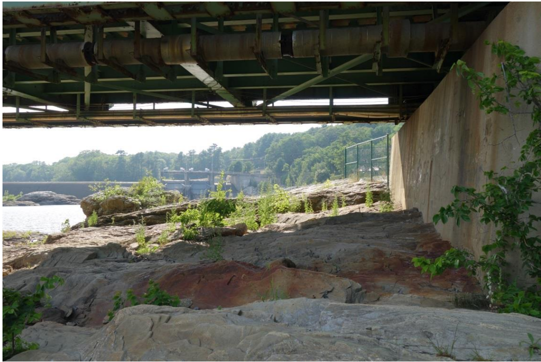
3.15 Existing Topsham abutment looking west
