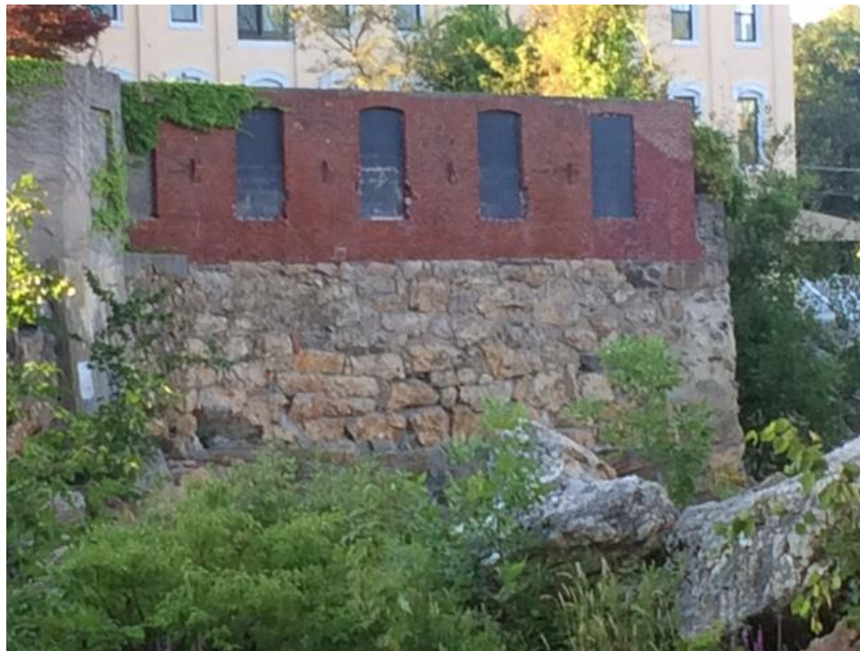
4.8 Old mill foundation now supporting Bowdoin Mill parking lot.
