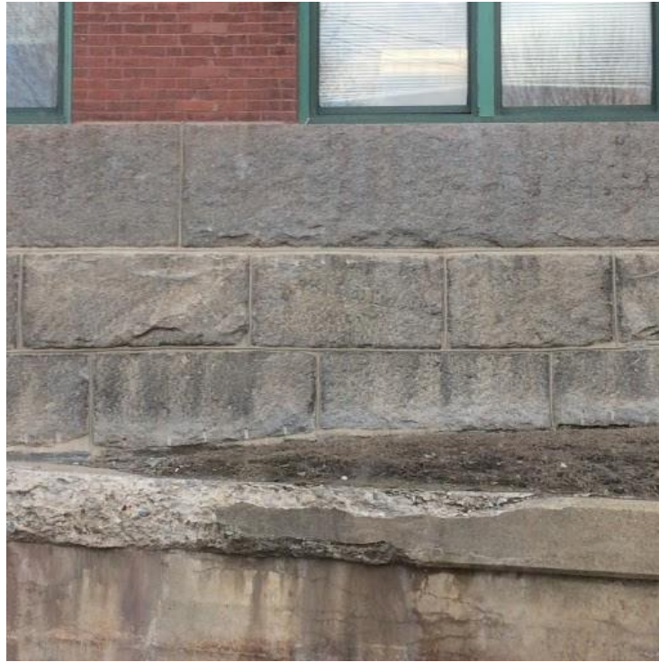
4.6 Cabot Mill Foundation, Brunswick
