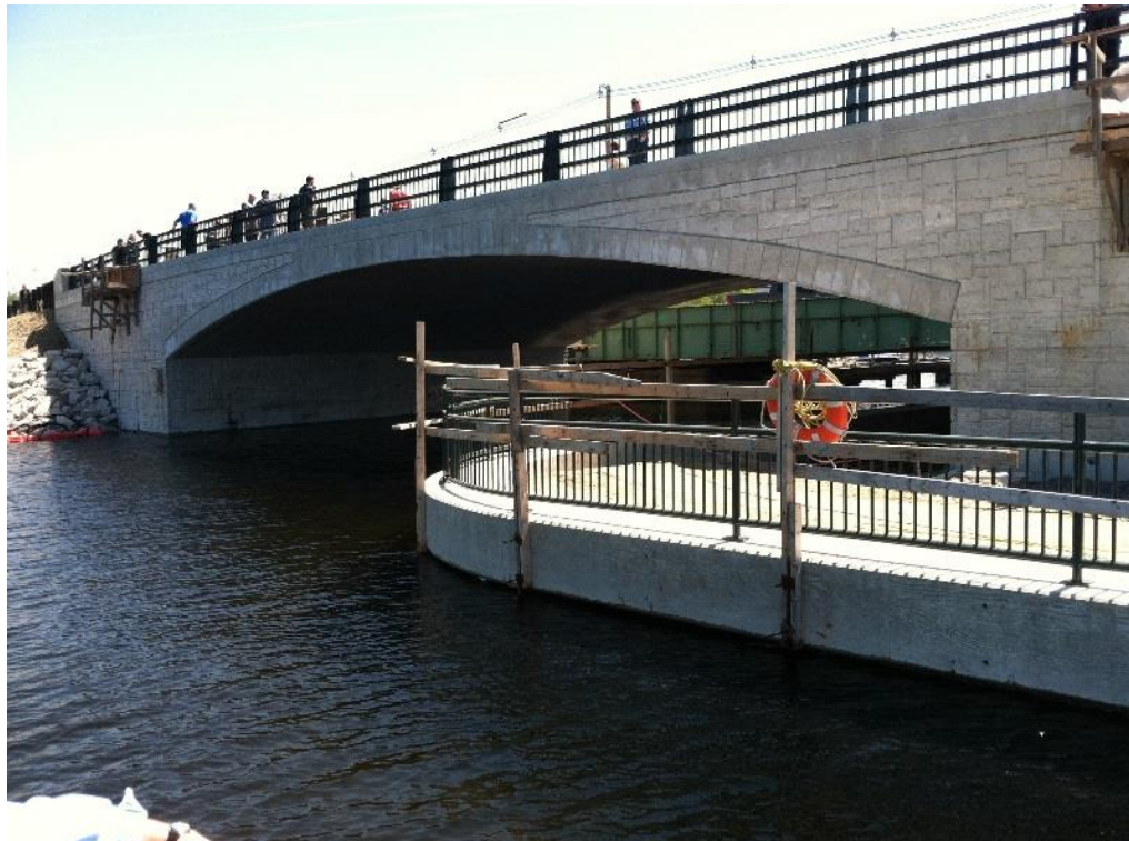
3.16 Pedestrian underpass example: Naples Causeway, Maine
