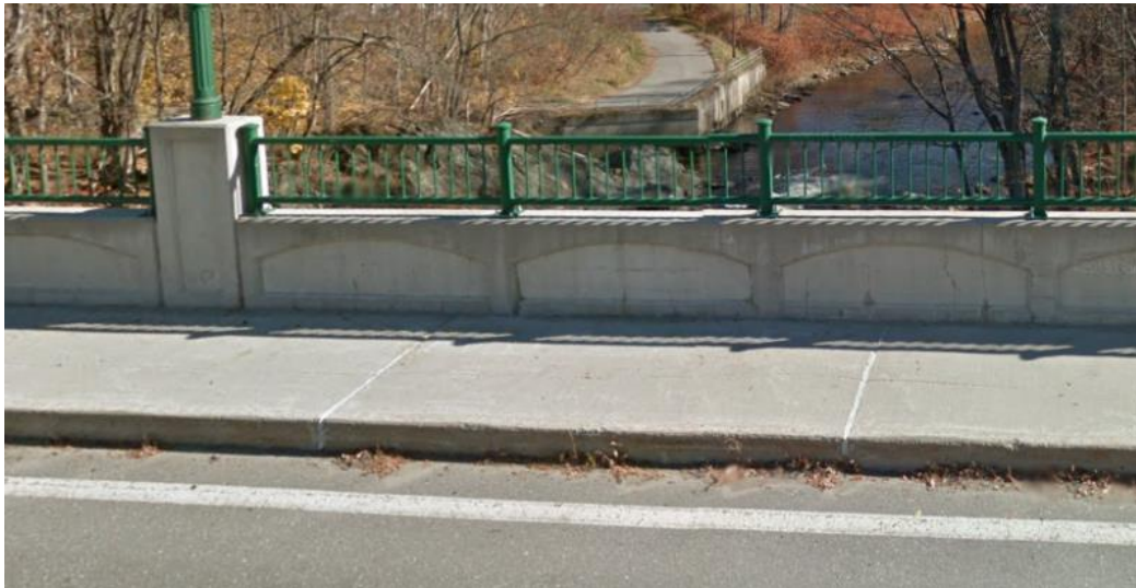
2.1 Railings inspiration: Saxons River Bridge, VT
