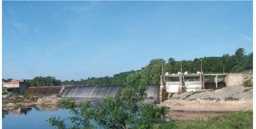
3.12 View upstream from Topsham Overlook
