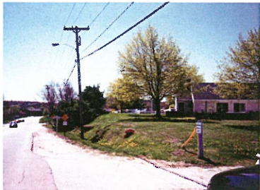
5. Congress Ave. looking south toward Centre Street intersection. Use existing pavement for bike lanes and construct sidewalk on right.
