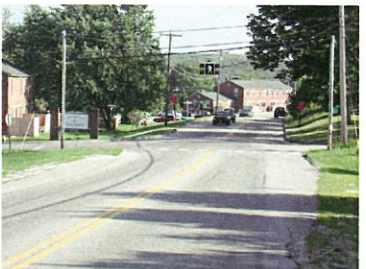
6. Congress Ave. looking south toward Centre Street intersection. Use existing pavement for bike lanes and construct sidewalk on right.
