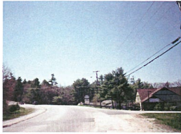
1. Congress Ave. looking west. Pavement widening required for bike lanes. Construct new sidewalk on right side.
