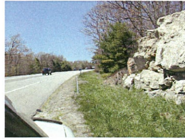
5. Pathway adjacent to Route one would require, stormdrain, guardrail, & protective fencing in this pinch-point area.
