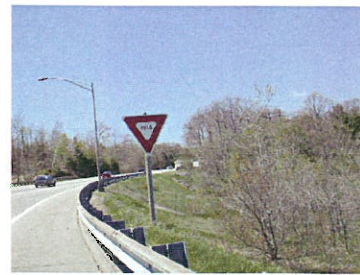
3. Proposed pathway location at mid slope. Minimum of 15' from guardrail.
