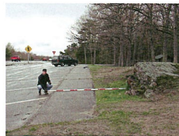
11. Minor blasting may be required to locate pathway and 5' buffer at rest area.
