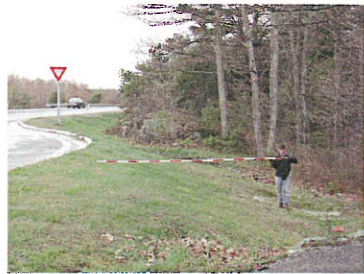
1. Fill and a culvert is required to continue pathway and maintain drainage
