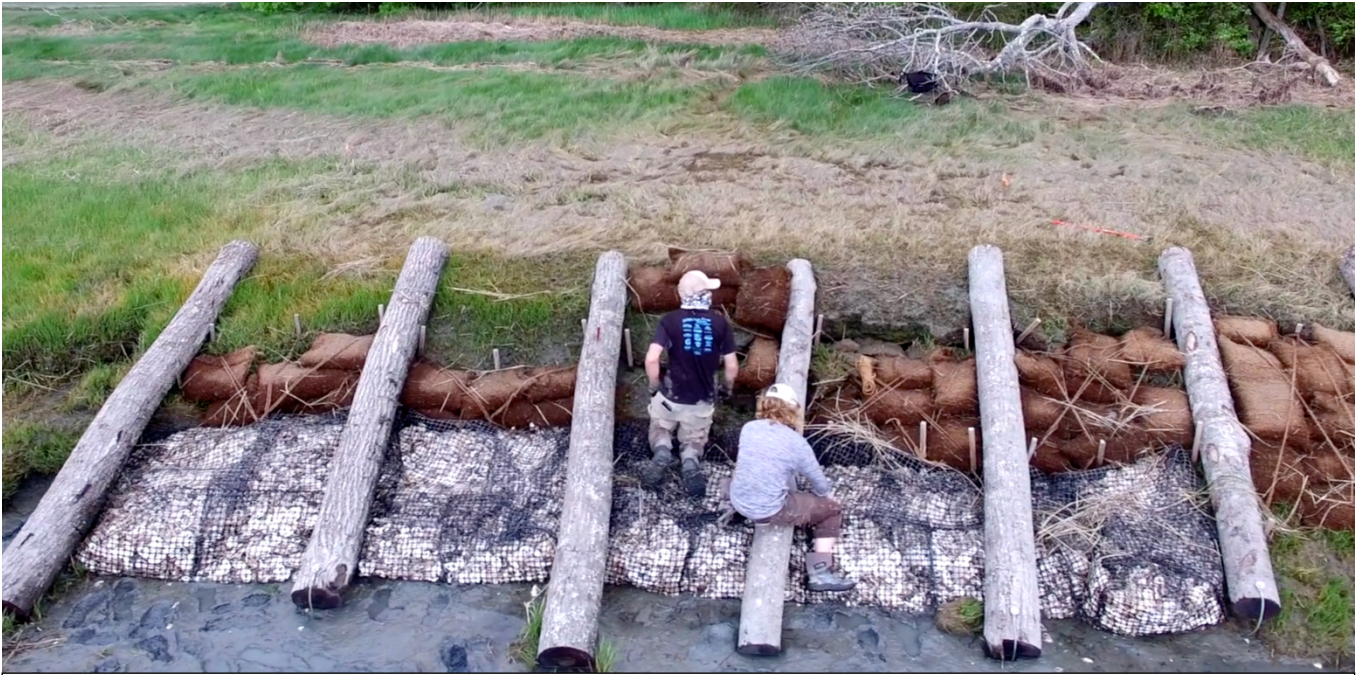
Shoreline Conservation Project at Maquoit Bay using oyster shells in coir fabric bags along with tree runners.
