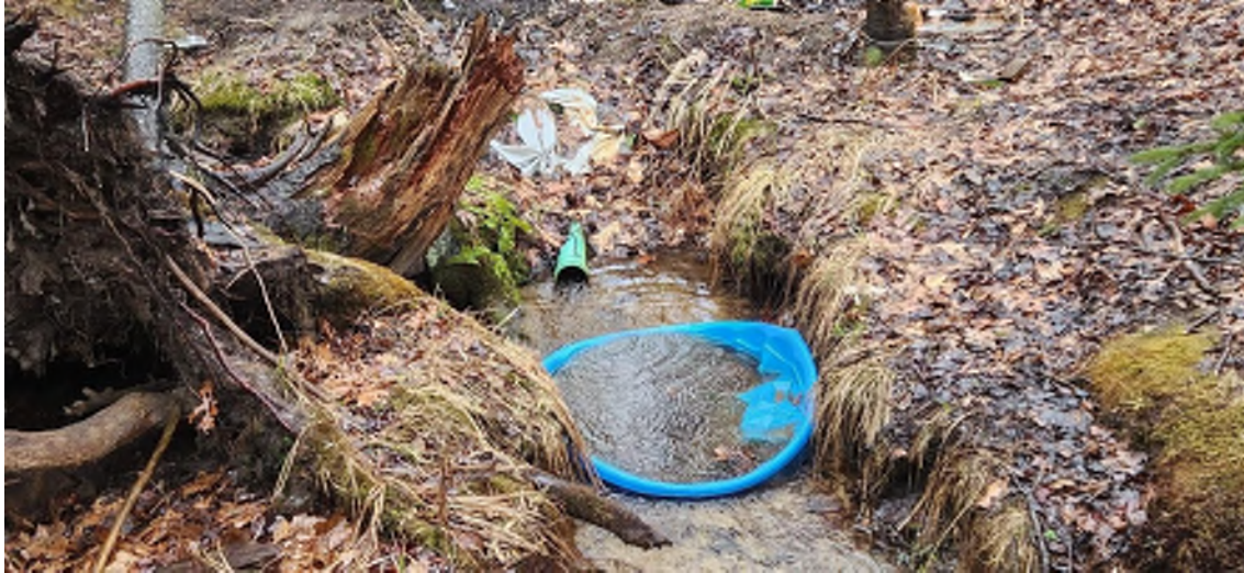
Photo 24: Drainage ditch with plastic culvert pipe within Wetland #4
