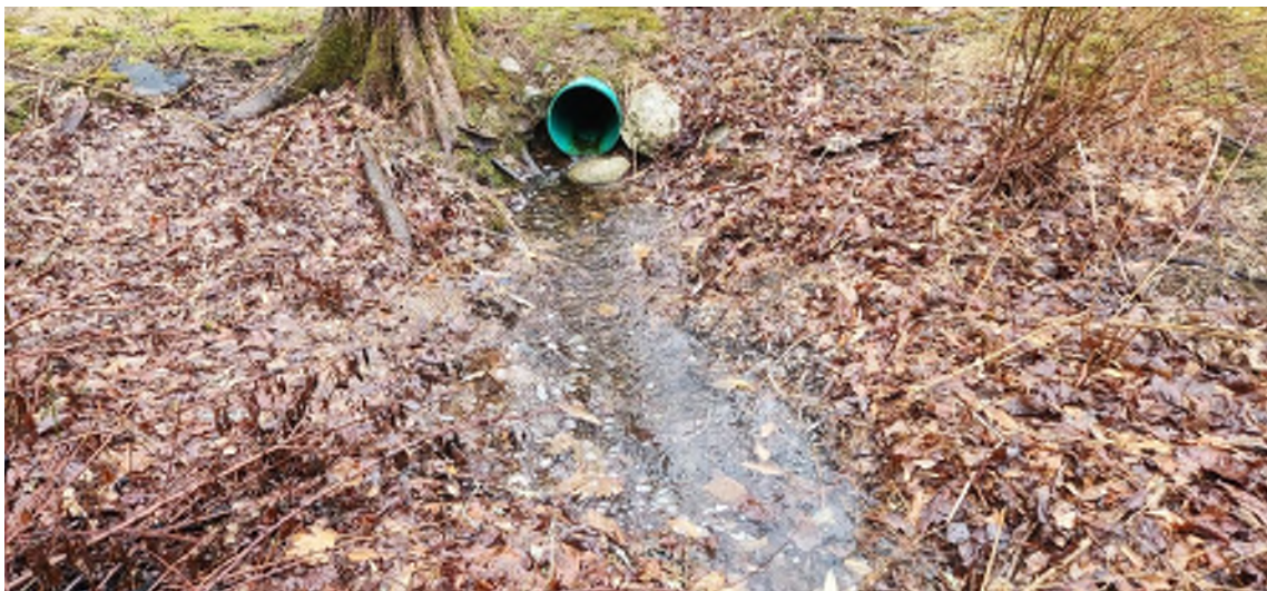
Photo 9: A culvert pipe from an abutting lot directs drainage into Wetland #4.
