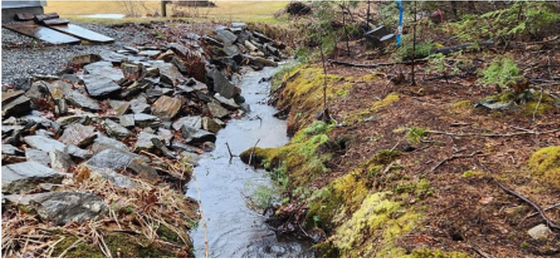
Photo 25: Rock-lined drainage ditch segment within Wetland #4
