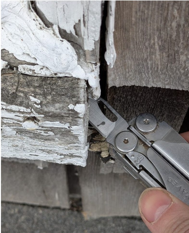
Figure 6: Rot on opposite bottom corner
